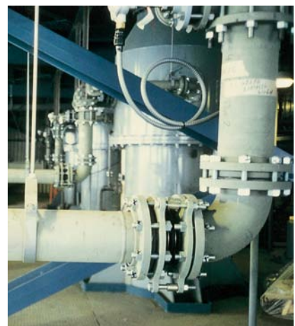
STENFLEX® type P1 in disposal pipes for chloro-electrolysis
